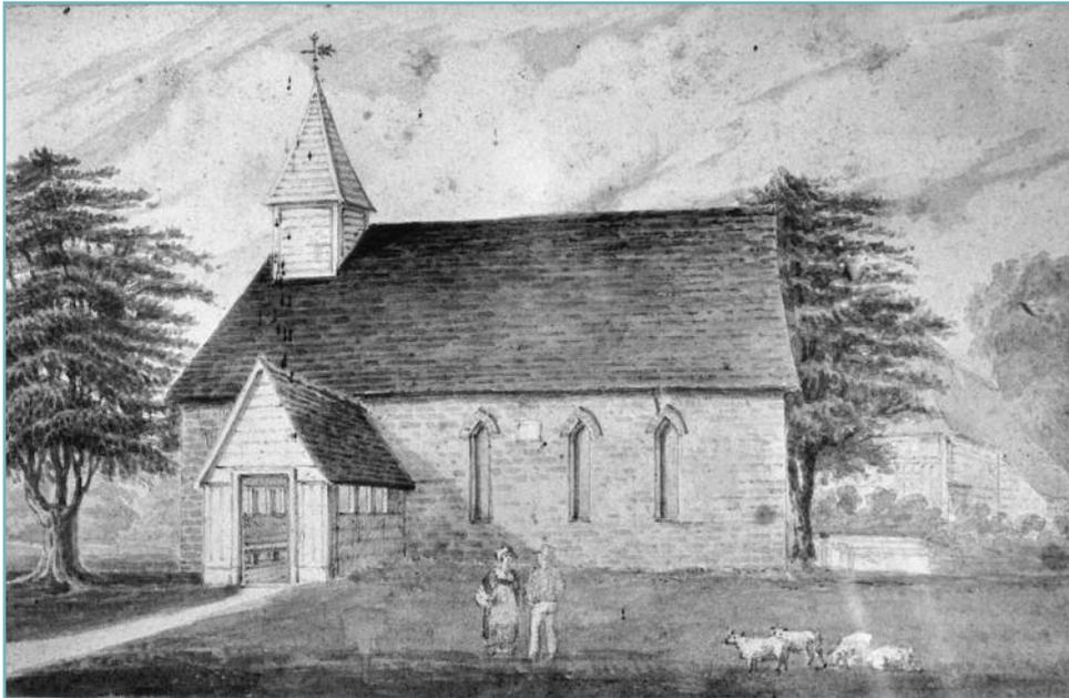
13th-century, church. The chancels of both buildings went to the edge of a disused chalk pit (later filled with spoil when the M2 was constructed nearby). This led to large cracks appearing in 1922 and the subsequent rebuilding of the east and south chancel walls. The list of rectors starts in 1313, although it is incomplete.
