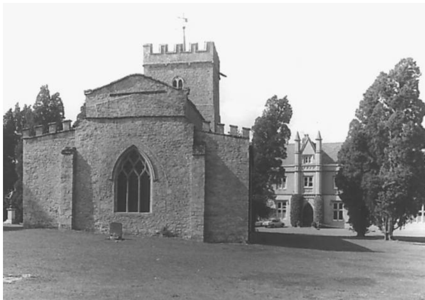
Church and Manor House
