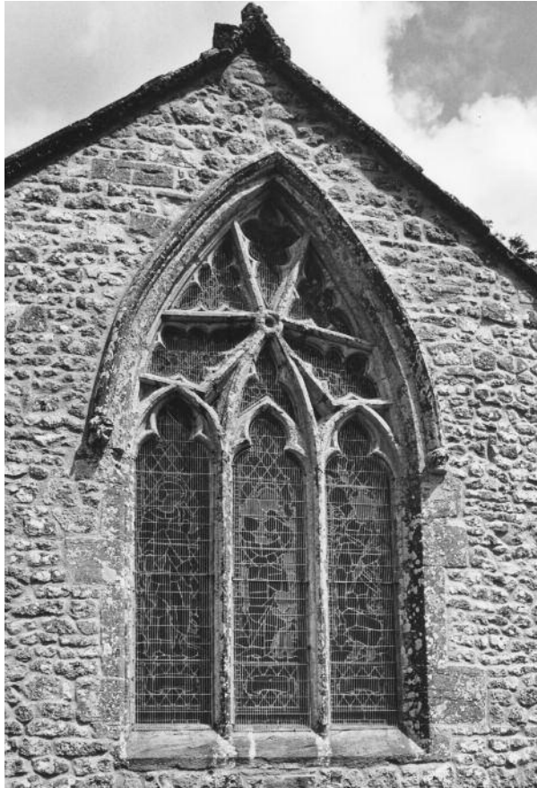
South window c.1300 of south transept, with its unusual tracery (CHRISTOPHER DALTON)
