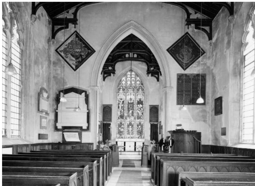
Interior looking east (ROYAL COMMISSION ON THE HISTORICAL MONUMENTS OF ENGLAND)
