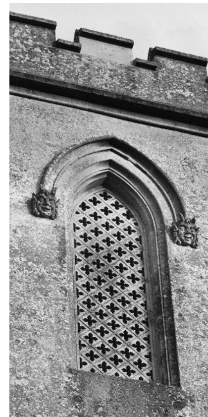
Belfry window showing the screen-like infill borrowed from mediaeval West Country churches (CHRISTOPHER DALTON)
