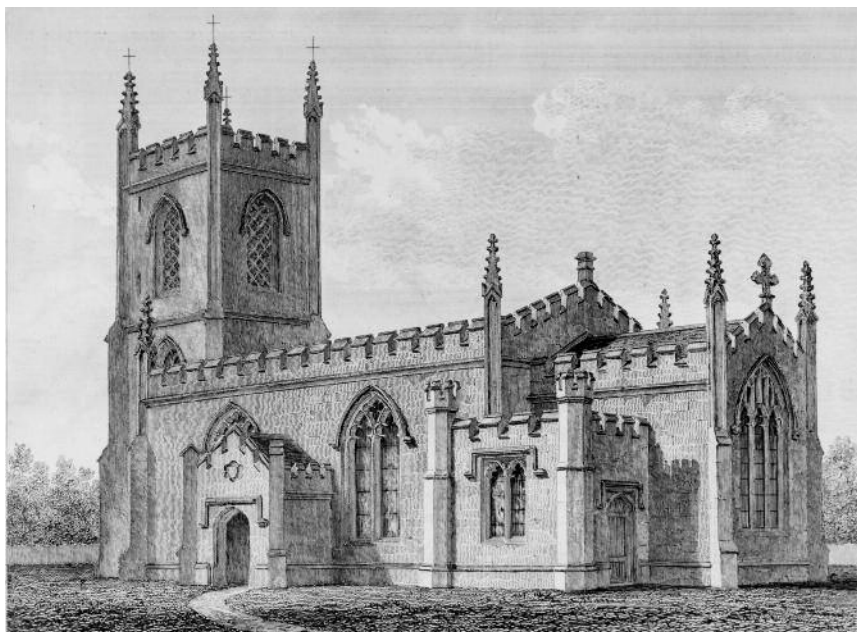
The new church
