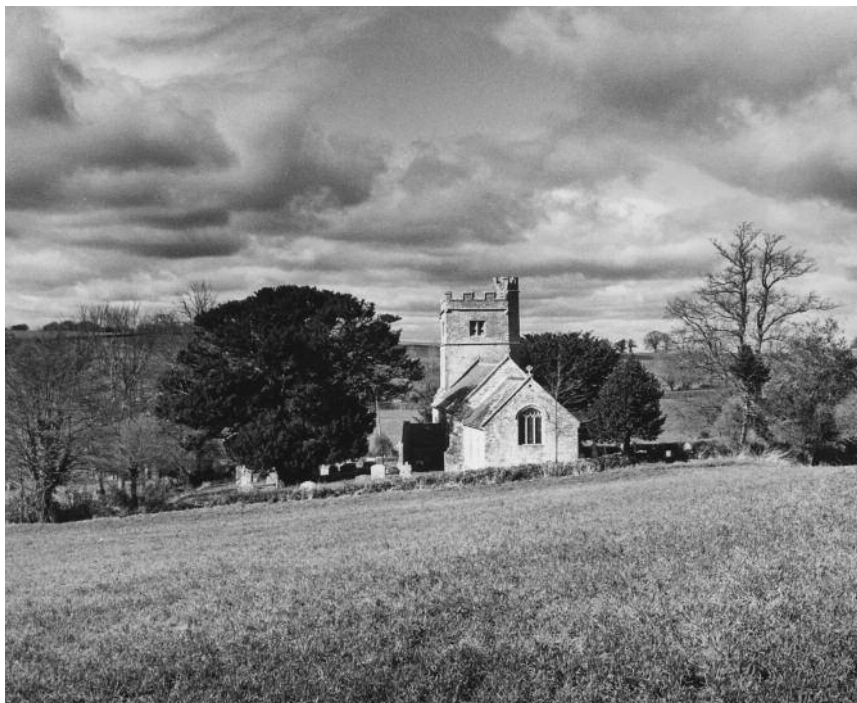
Exterior from the east
