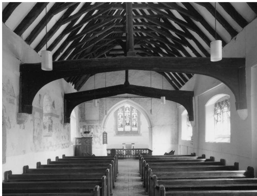
Interior looking east
