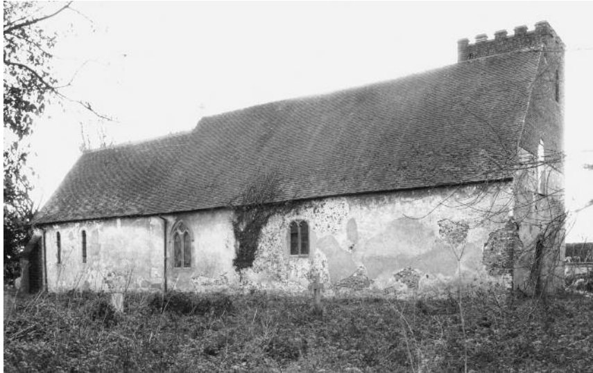
North side of the church
