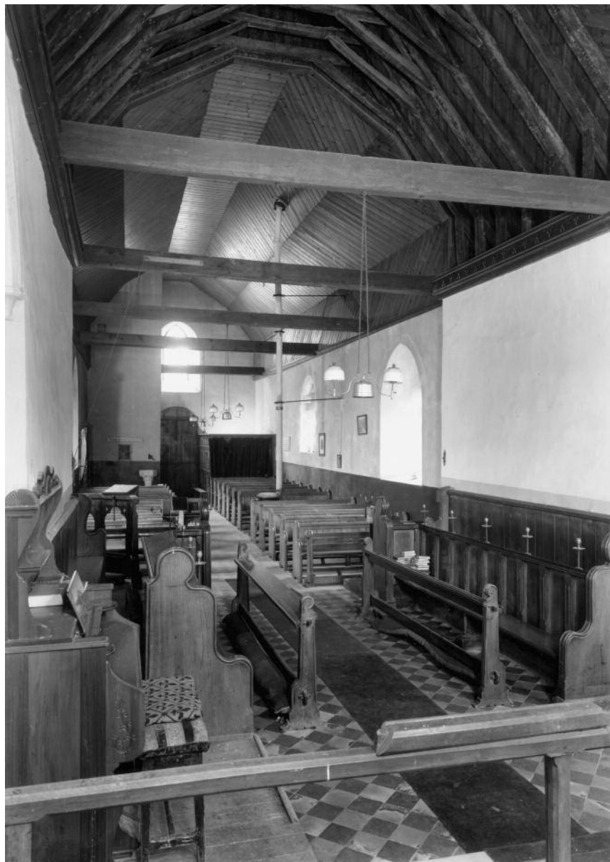
Interior looking west in 1972
