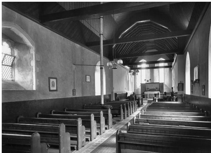
Interior looking east in 1955
