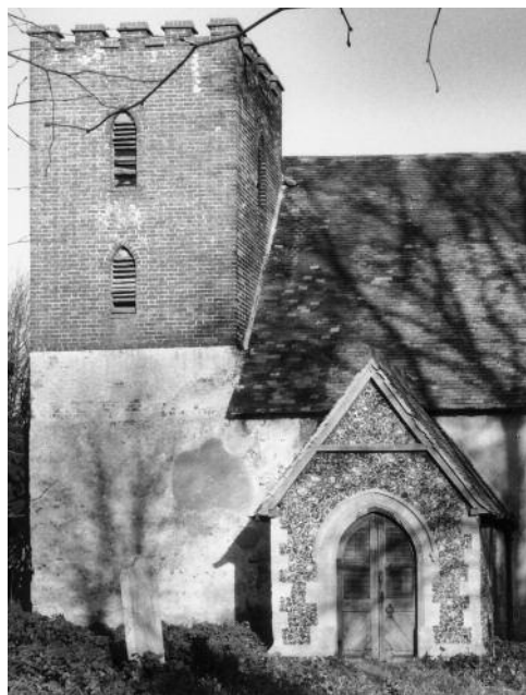
Tower and south porch (CHRISTOPHER DALTON)
