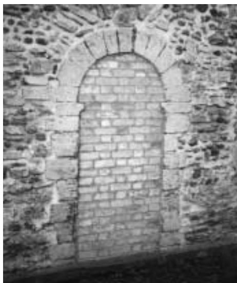
The original Saxon doorway is now blocked up.
